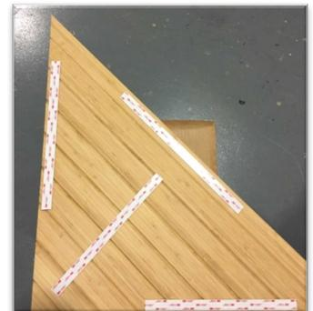
Please carefully note: The initial placement of the Fractal panels must be carefully performed to make sure all panels are square to a snap line, your wall, or the sheathing edge line, as appropriate. All subsequent Fractal panels will be installed to the right of this line, so it is of utmost importance that the initial panel be square and straight in its initial application.
