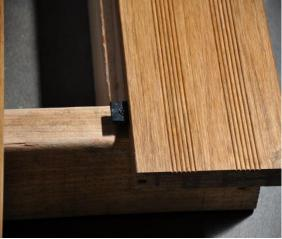
Insert a clip in the slot and slide in a screw and drive the screw in till it just touches the top of the clip. (see picture) The clips should be just level, do not over tighten or they will by slanted, amking ti difficult to side the next board in place
