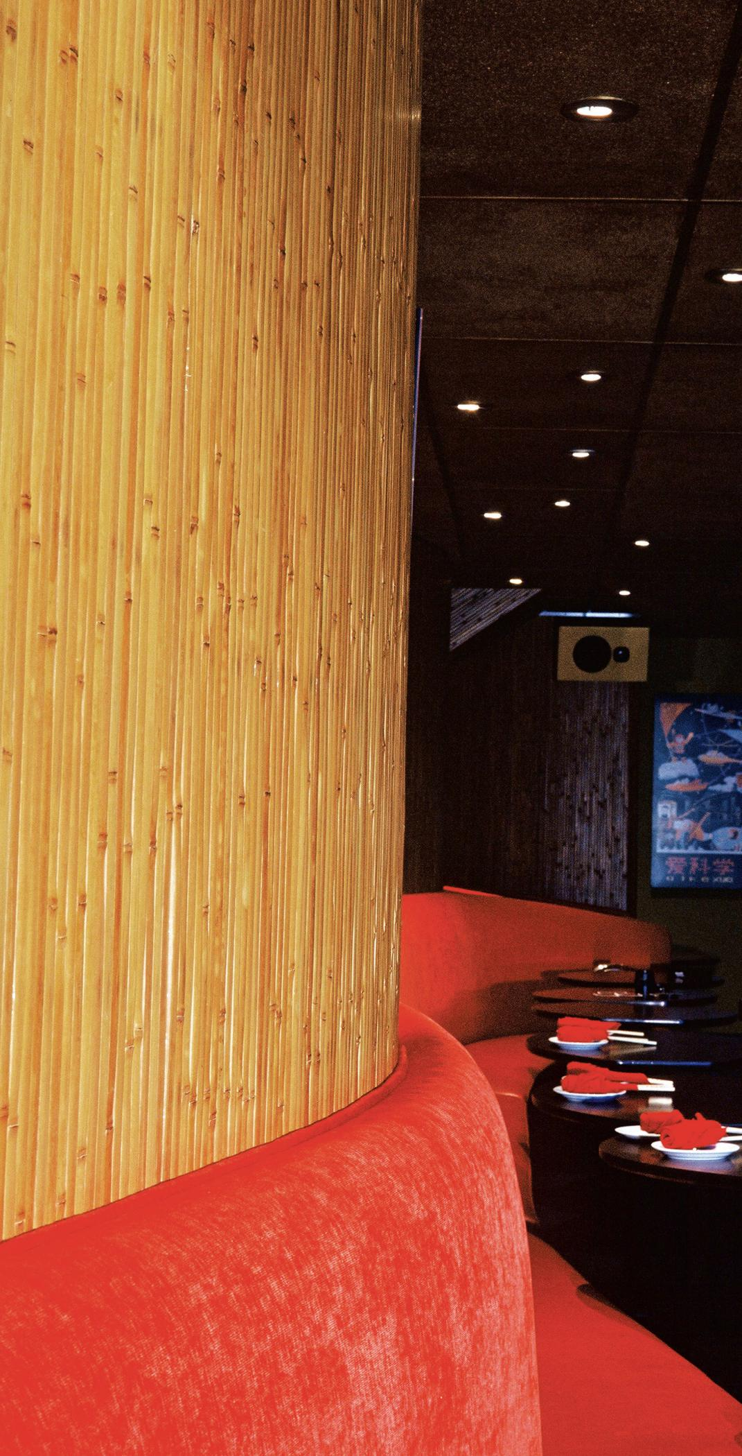
**Plyboo tambour paneling** is constructed of bamboo strips that are precision milled and applied to a thin fabric backing.
